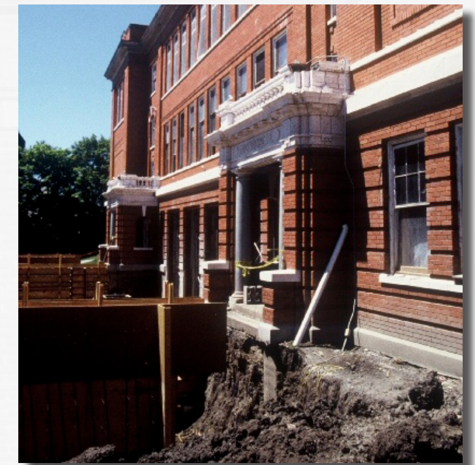
Construction of new plaza begins in 2001
