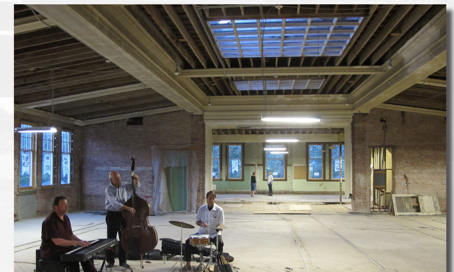
Removal of dropped ceiling reveals skylights over the former third floor auditorium
