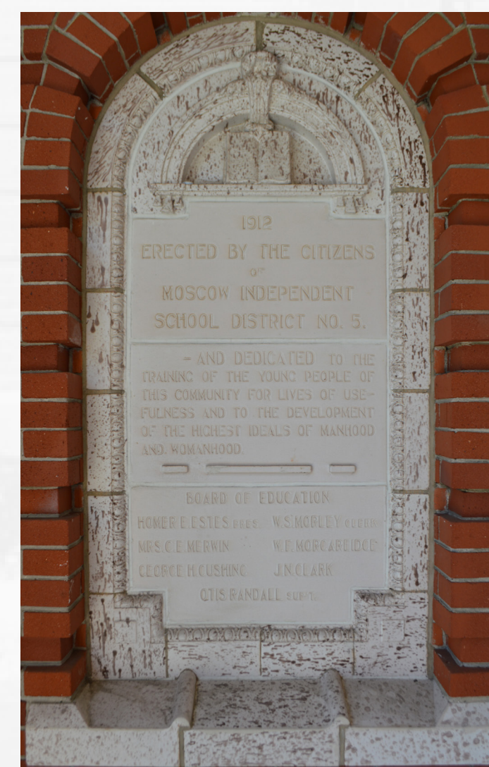
Dedication plaques mounted in south facing entry porticos
