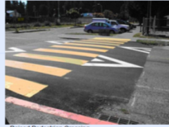
Raised Pedestrian Crossing
