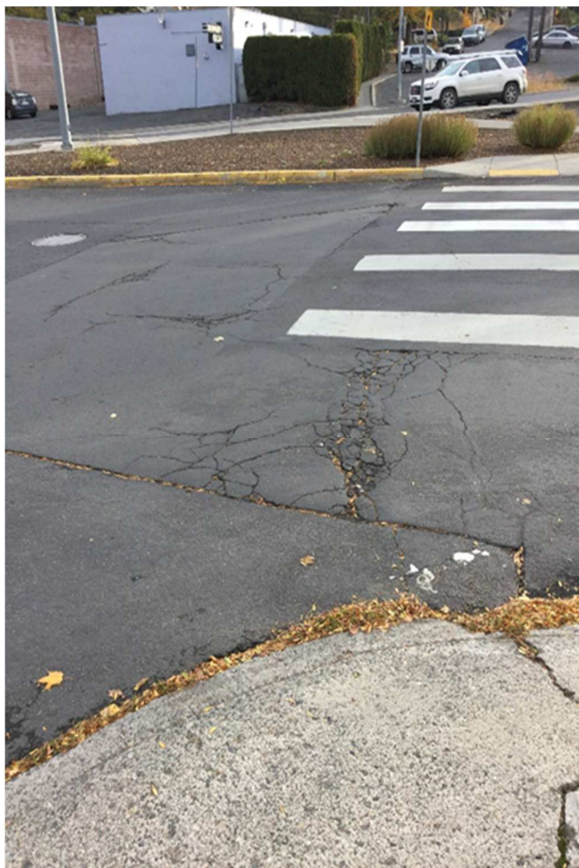
Figure 4 Example Infrastructure Condition Photograph
