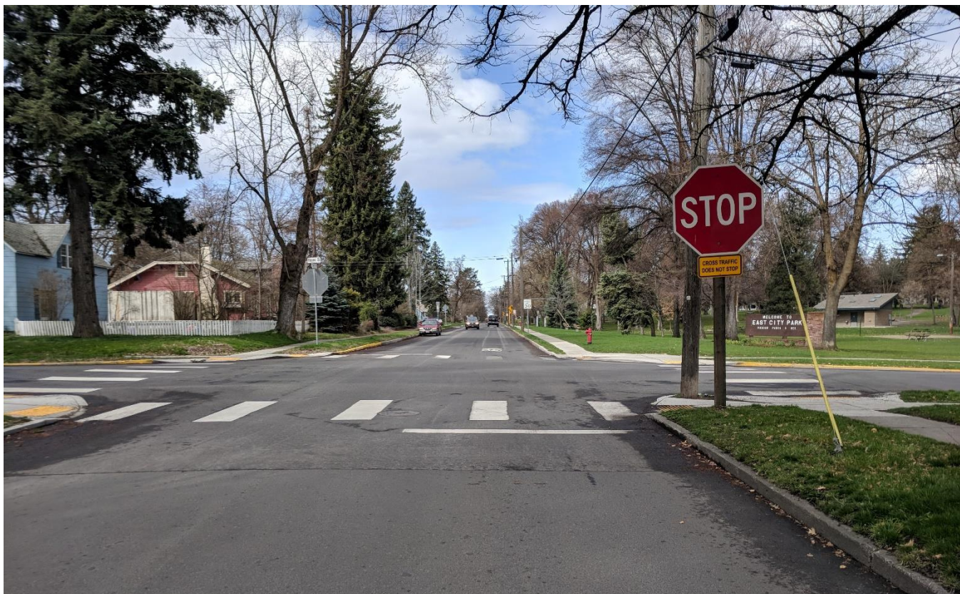
Figure 7. 3 rd Street looking west from Hayes Street
