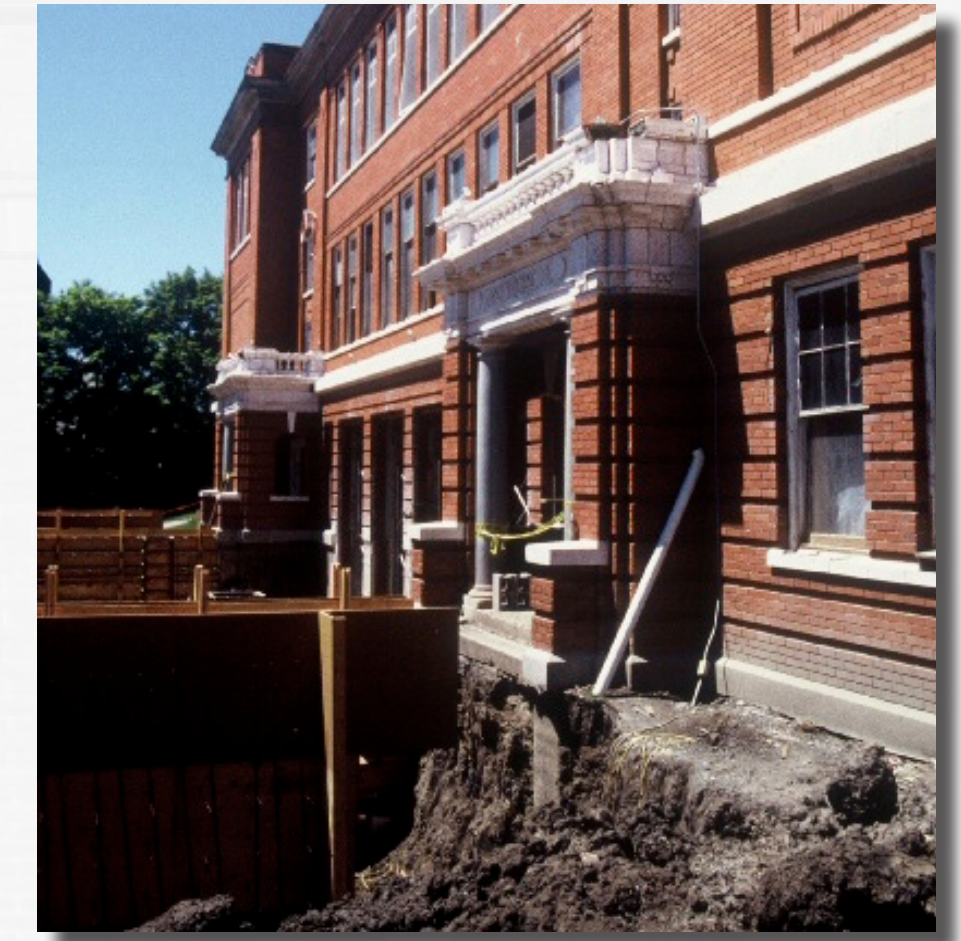
Construction of new plaza begins in 2001
