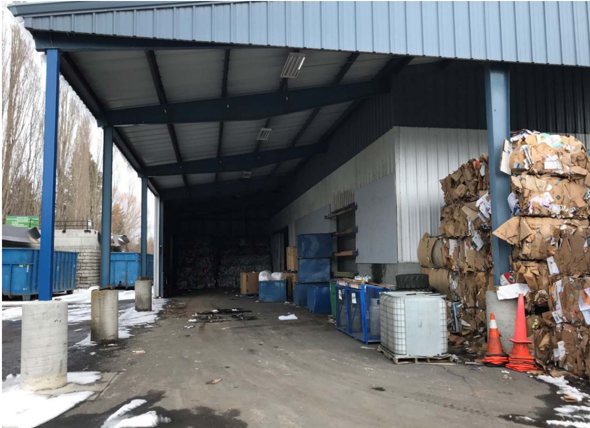
Exhibit 9. View of the Covered/Dry Storage Area Looking North (West Side of Main Building)
