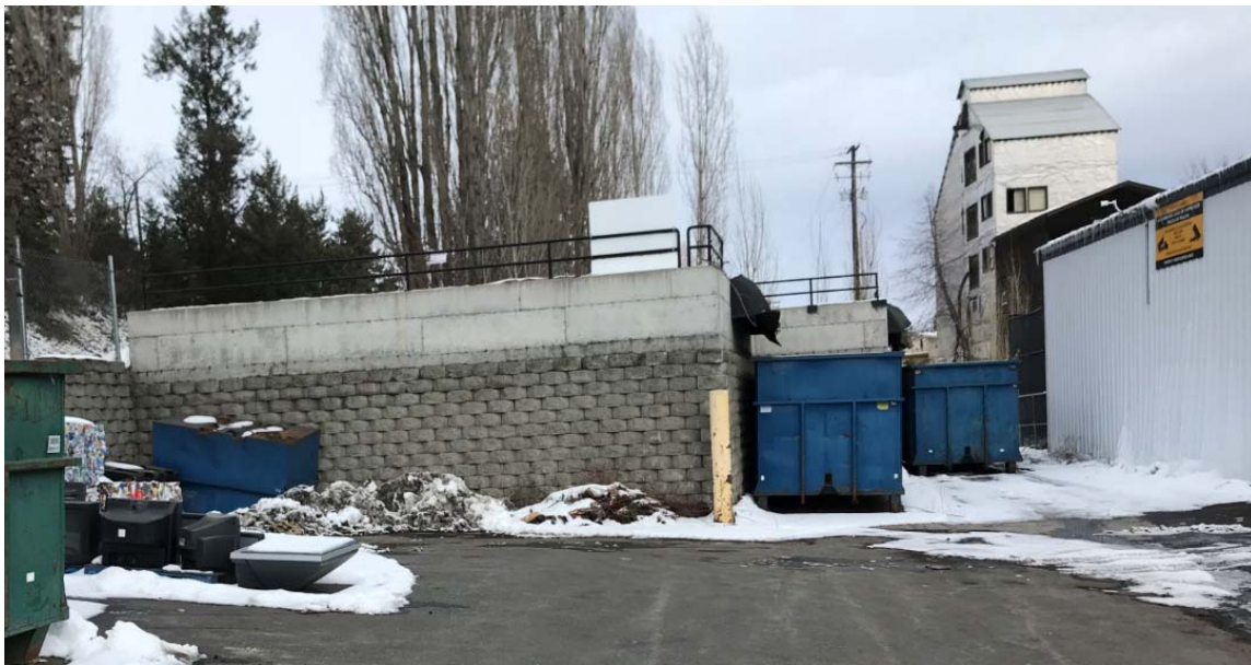
Exhibit 10. Yard Waste Drop-Off Area (Z-Wall) Looking North at Lower Level
