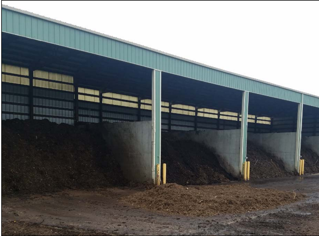
Exhibit 6. Static Pile Composting Operations at the SWPF
