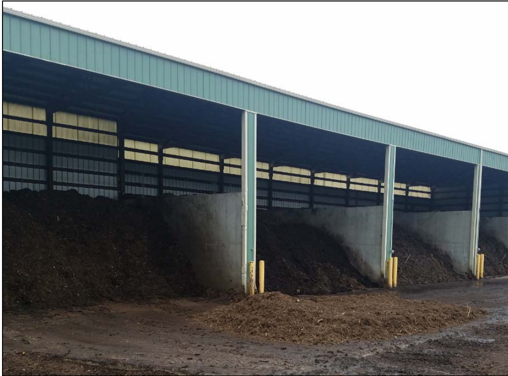
Exhibit 6. Static Pile Composting Operations at the SWPF
