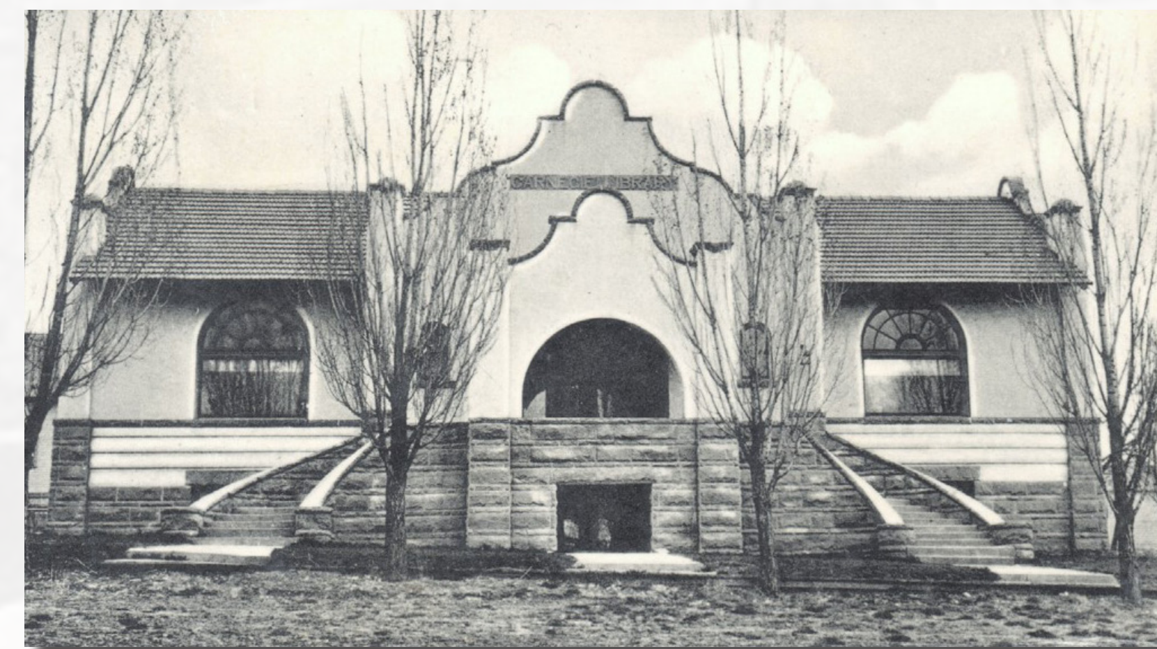
West facade showing original Mission Revival style
