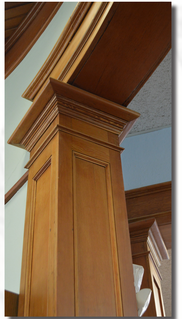
Millwork detail in the former entry lobby of the original 1906 structure
