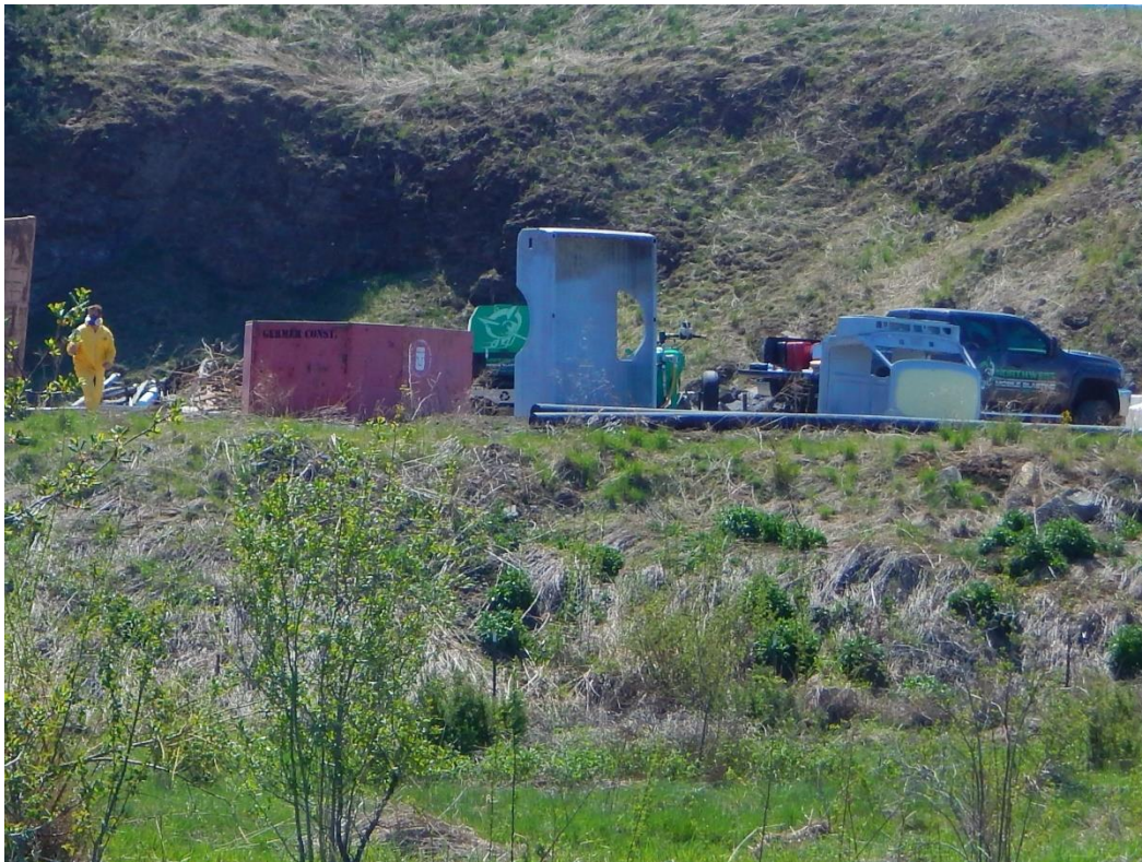
Figure 6 Sand Blasting in rock pit
