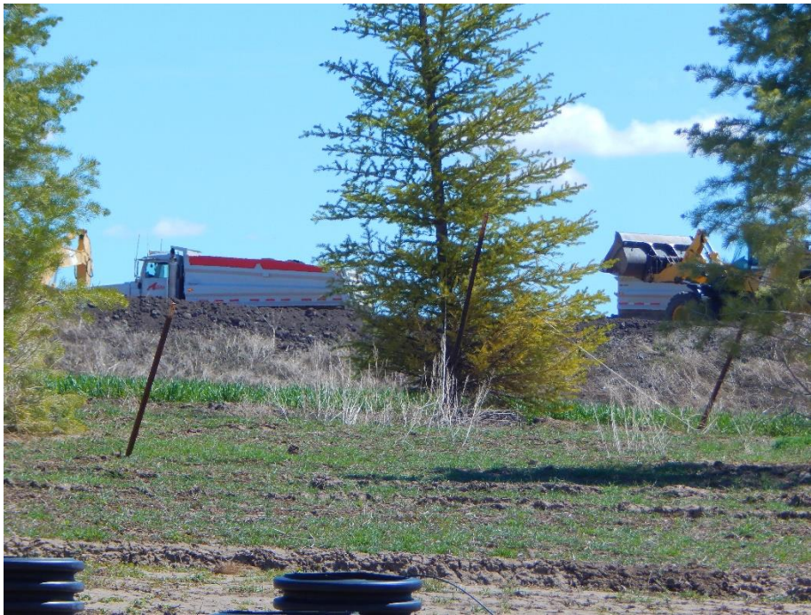
Figure 10 Atlas truck and trailer loading black dirt
