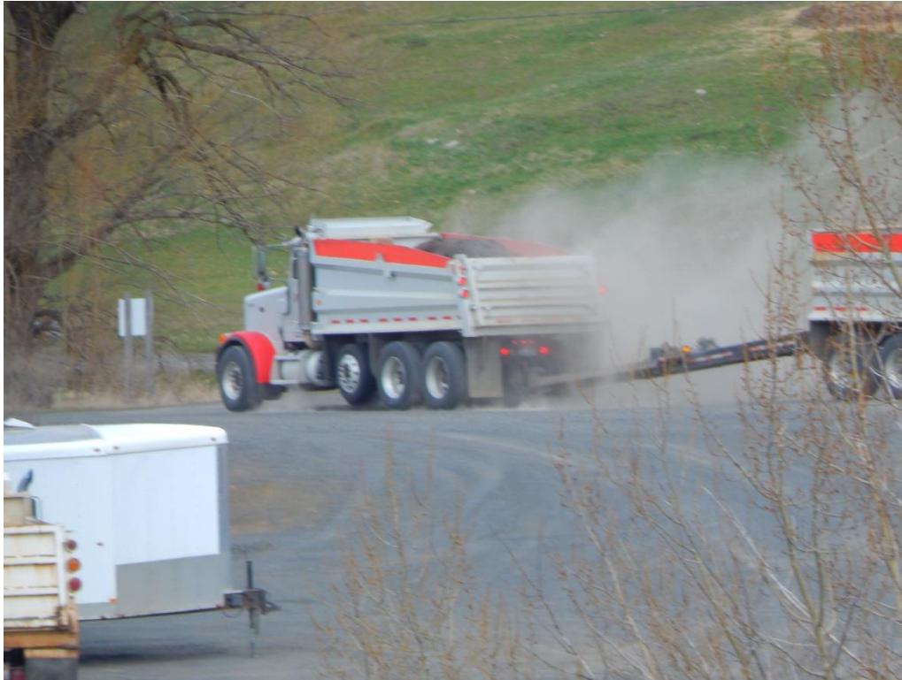
Figure 5 Truck causing dust while hauling out black dirt
