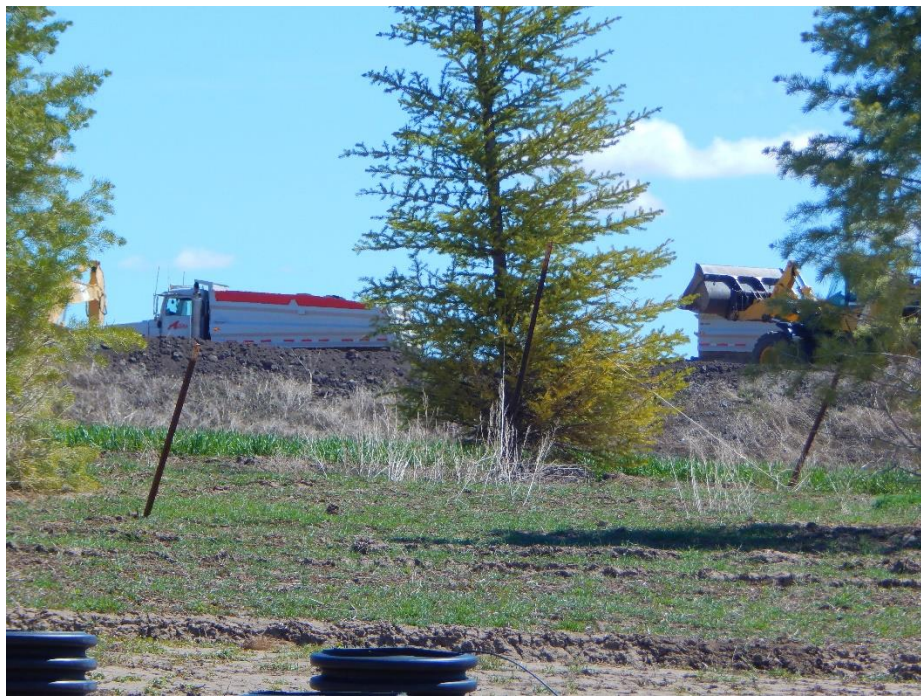
Figure 10 Atlas truck and trailer loading black dirt
