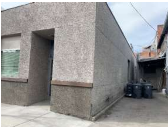
Rear View – Northeast Corner
