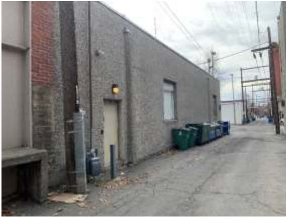
West View – Public Alleyway
