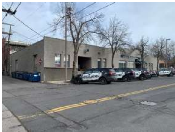
West Side/Front View – Southwest Corner
