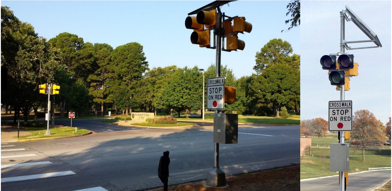
Figure 9. Potential Pedestrian Hybrid Beacon (HAWK) configuration for use at 3 rd Street and Mountain View Drive.
