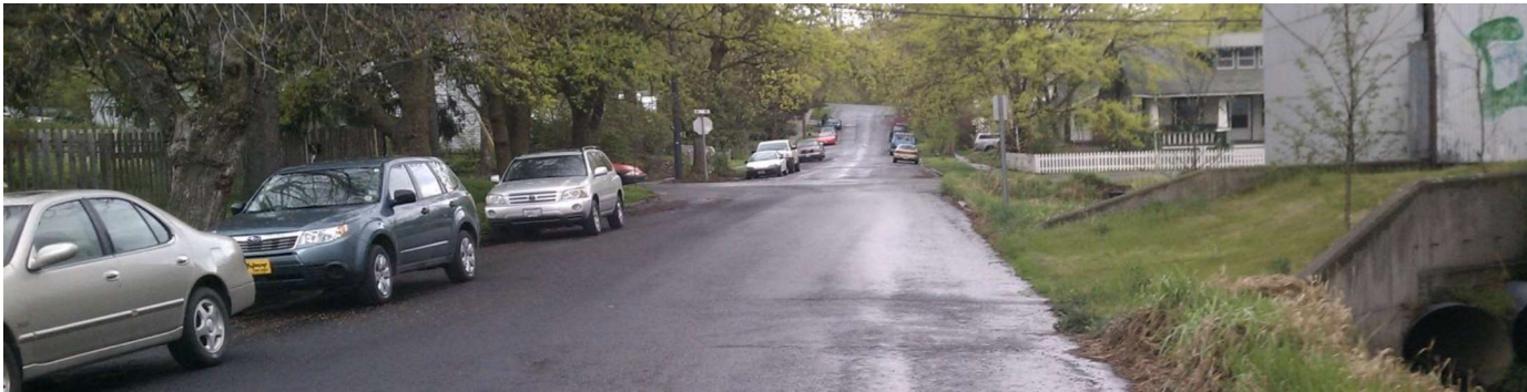
Asbury Street is a key university access route for students, faculty, and staff, but offers no sidewalks and limited separation from traffic. Image from Nelson\Nygaard
