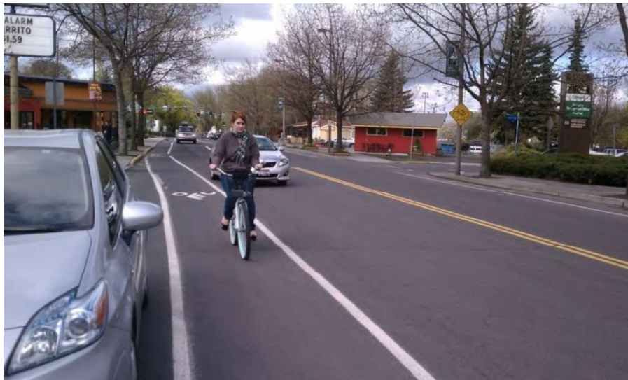
At five feet wide, the Sixth Street bike lane is relatively well designed. However, high parking turnover increases the chances of open door, or "dooring", hazards.
