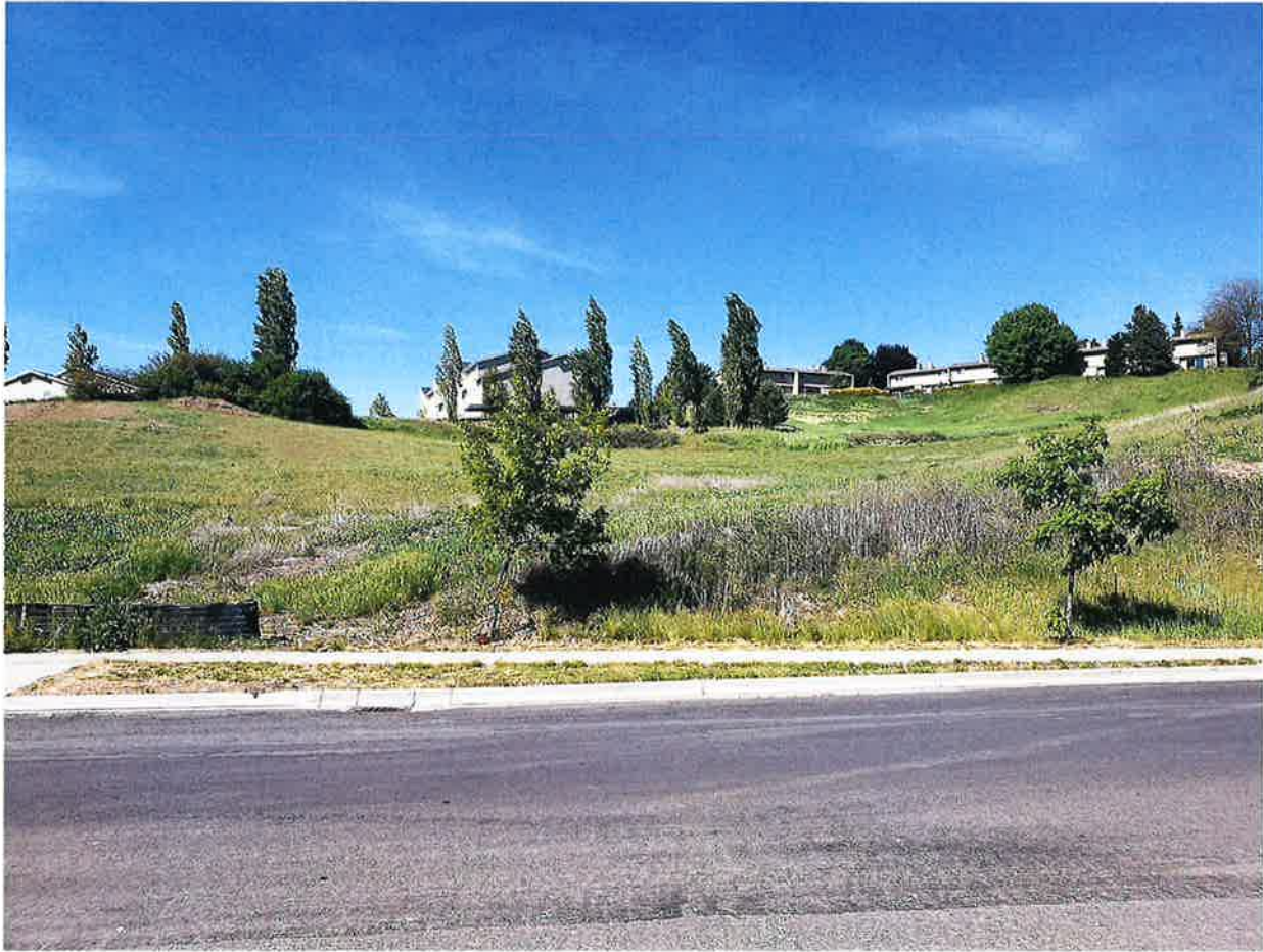
Photograph 1. Indian Hills Booster Pump Station Site
