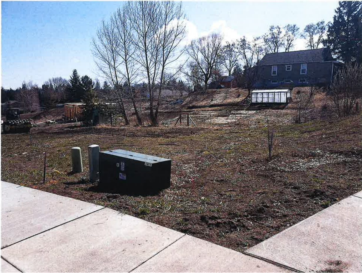
Photograph 2. Ponderosa Booster Pump Station Site
