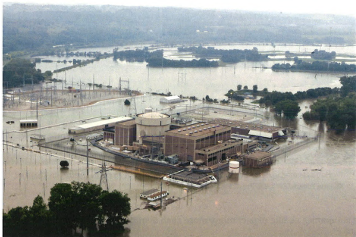
Flooding in 2011 forced the Fort Calhoun nuclear power station near Omaha to shut down for years. Nati Harnik/Associated Press
