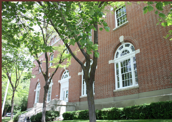
Figure 2.2: Moscow City Hall (former Post Office and Federal Courthouse)
