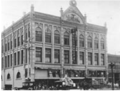
McConnell Maguire Building
