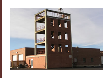
Station No. 2 1300 East White Avenue
