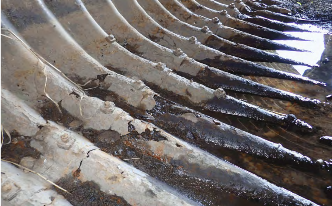
(240-Culvert CS4) South barrel: laminar rust with 100% section loss.
