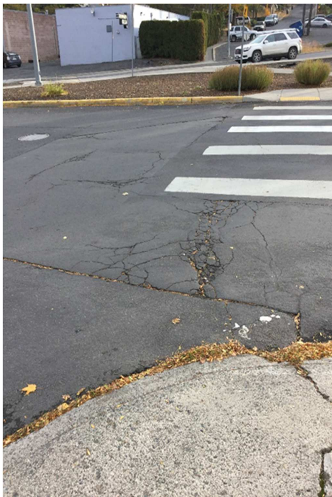
Figure 4 Example Infrastructure Condition Photograph
