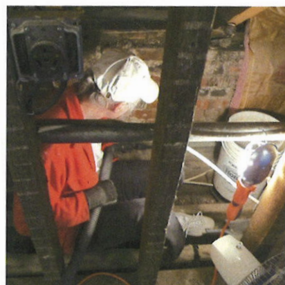
Brick work in the second story wall.
