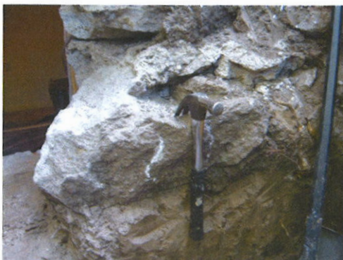
Close-up of the foundation granite.
