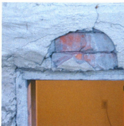
Brick work above the basement window.
