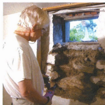
Nels Reese with jackhammer.
