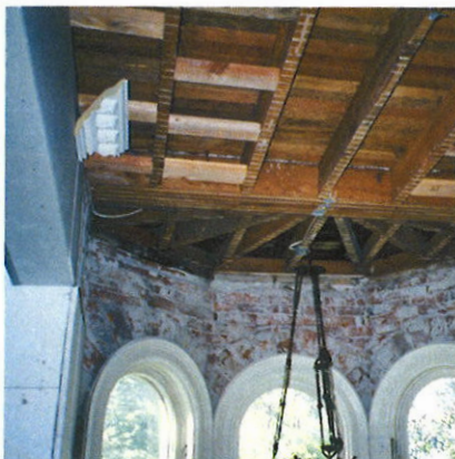
Dining room under re-construction.
