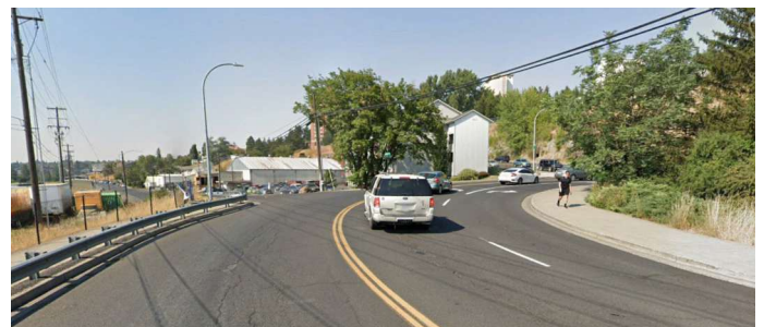
Bishop Blvd and SR270 Intersection.
