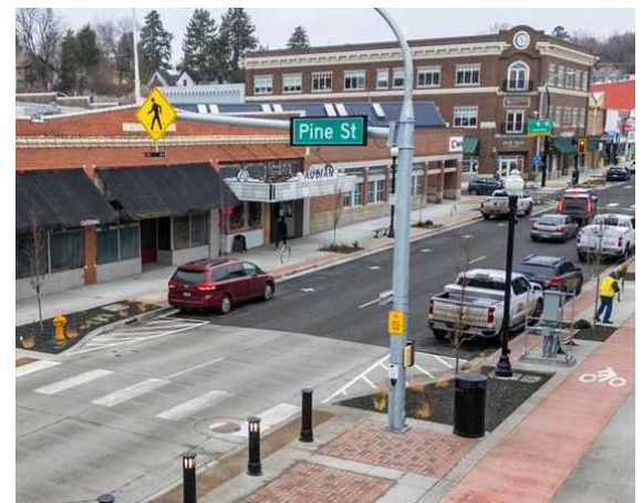
Revitalization of Pullman's Main Street in 2024 introduced traffic calming measures—like curb bulbs, road diet, narrower lanes, and a speed table—to enhance pedestrian connectivity and encourage trucks to use alternate routes.
