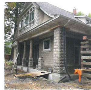
Aug 28 Columns saved
