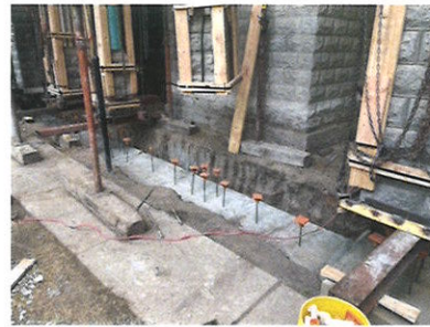
July 22 New Footings
