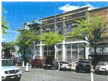
In progress work...
