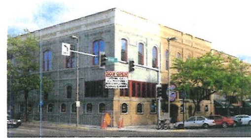
2010 Stucco finish and small windows
