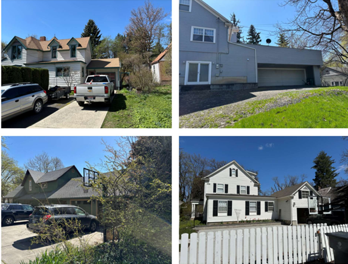
Fig. 2.2: Attached garages at 328 N Polk, 415 N Polk, 323 N Howard, 634 E B.
