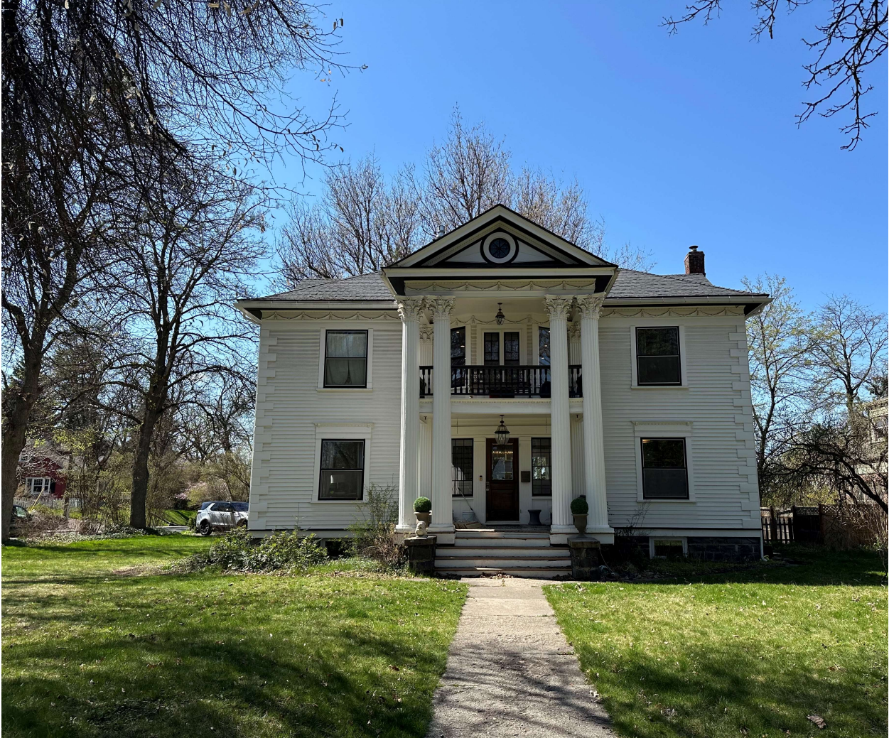
Fig. 1.1: Photo of front setback at subject property.
