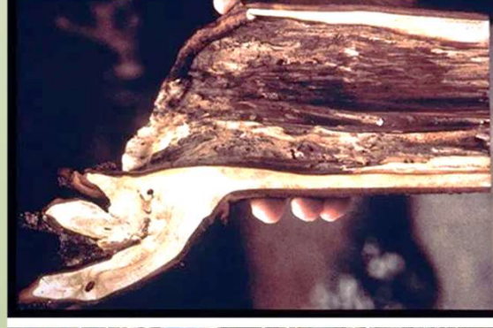
Significant decay can develop within the stubs.
