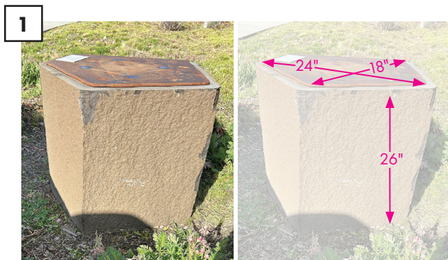
Basalt plinth with weld plate • 26" H x 24" L x 18" W Dimensions on weld plate are the longest sides of an irregular polygon.
