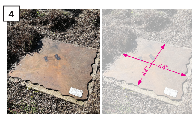
Ground plinth with weld plate • 44" W x 44" L
