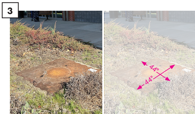
Ground plinth with weld plate • 44" W x 44" L
