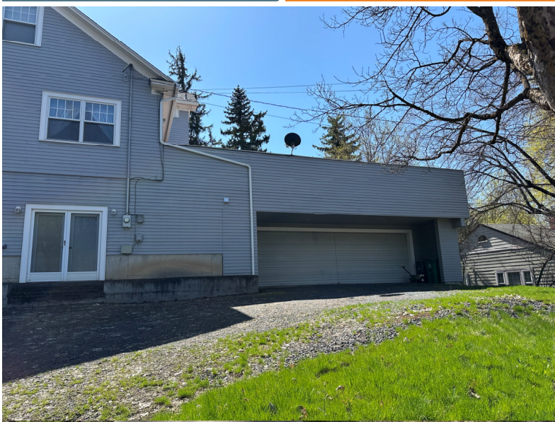
415 N POLK ST Attached garage at five feet from property line
