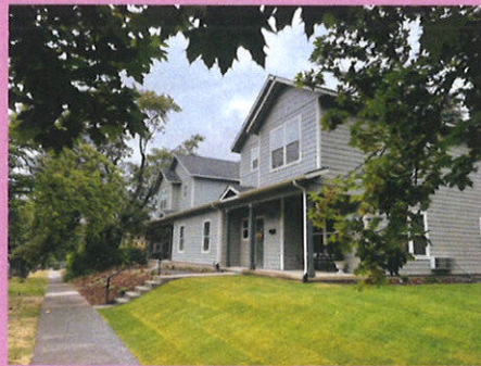
Completed duplex in July 2025
