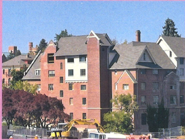
Completed roof on Sep 17, 2025
