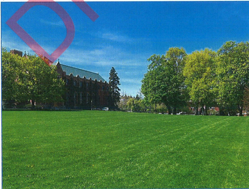
Photo 10: View of Administration Building (10LT52) and Art & Architecture South (10LT426) over Administration Lawn (10LT1472), Image by Nathan J. Moody, April 30, 2025.
