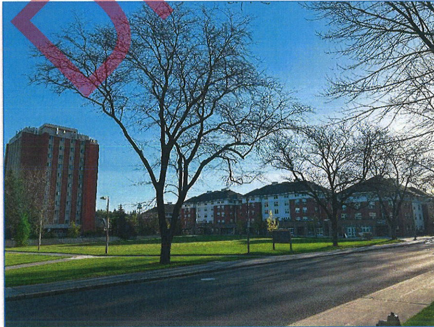
Photo 26: View of Theophilus Tower (10LT2301) and LLC Complex (10LT2276 – 2285) from Sixth St., Image by Nathan J. Moody, May 1, 2025.
