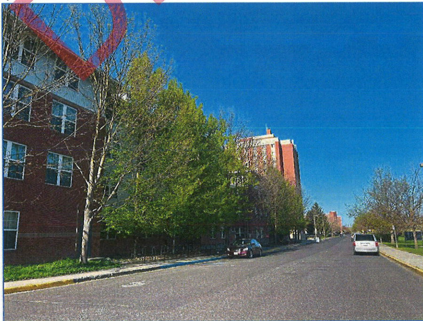
Photo 34: View of LLC Complex (10LT2276 – 2285) and Theophilus Tower (10LT2301) from Paradise Creek St., Image by Nathan J. Moody, May 1, 2025.
