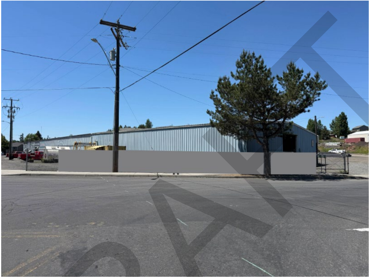
Mock-up of concrete wall to be built by the City of Moscow in 2026.
